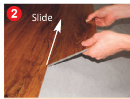
2 Slide Angle the second plank and align the interlocking strips
